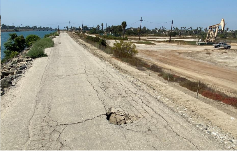
Levy asphalt sunken in
