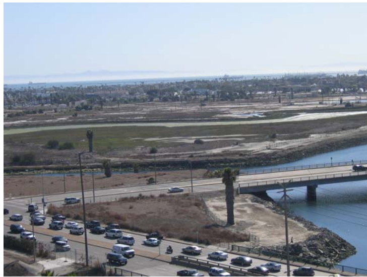
Figure 5.5: Steam Shovel Slough with Catalina Island in the background. Photo: Garcia, 2007
