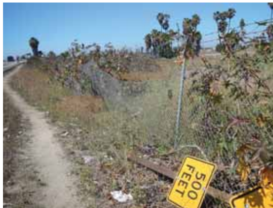
Figure 3 Collapsed fence needs immediate repair
