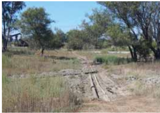
Figure 8. Exposed pipeline
