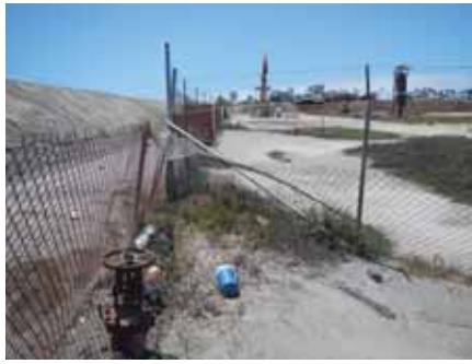
Figure 7. Collapsed fence
