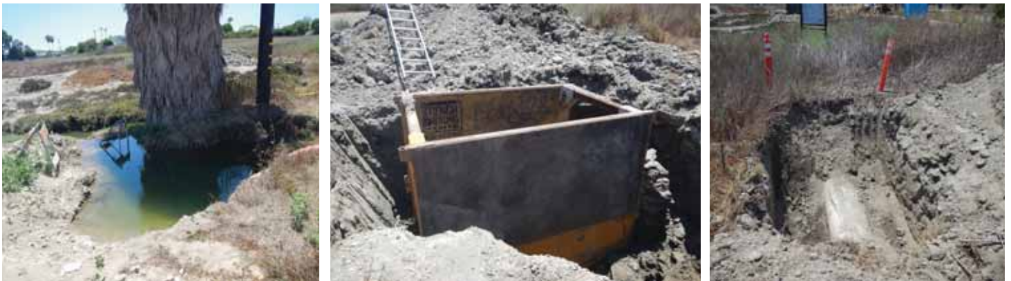
Figure 6. Three holes of Waterline excavation
