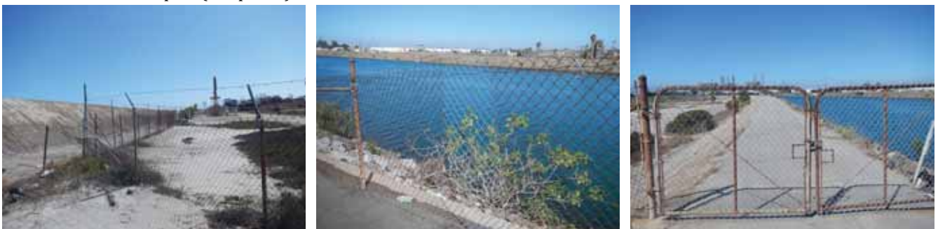
Figure 6. Collapsed fence (left) and fixed fences (middle, right)
