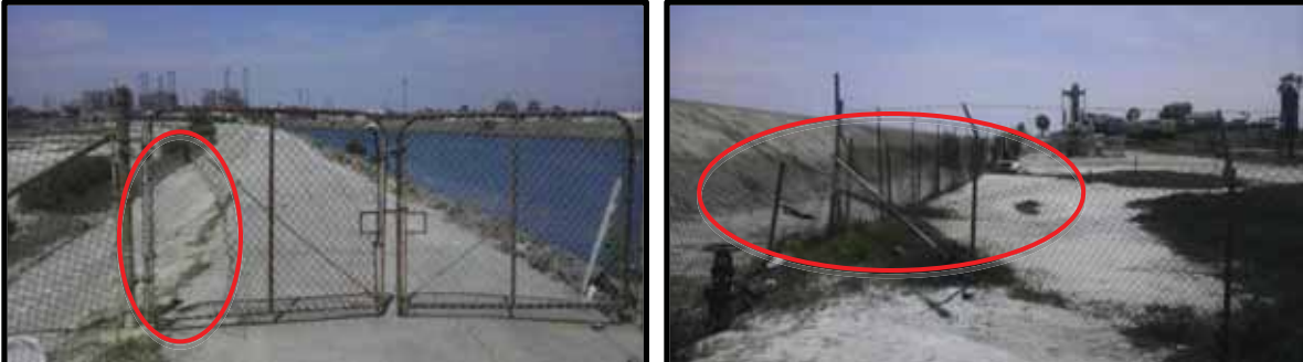
Figure 4 Hole in fence (left), collapsed fence (right)
