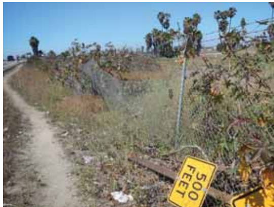
Figure 3 Collapsed fence needs immediate repair
