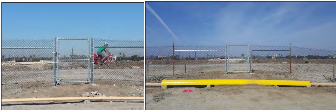
Figure 2. New Zedler Marsh gate before and after pipe cover.
