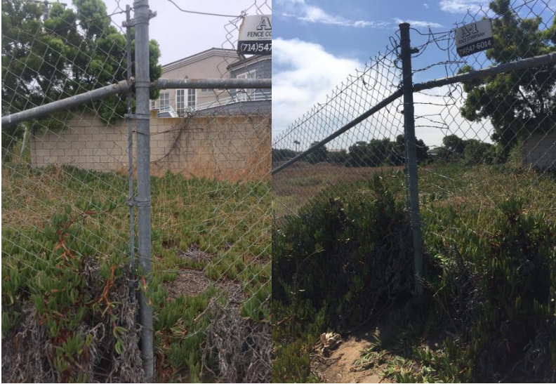
Fence Breach Patches
