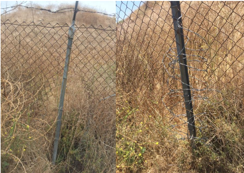
Fence Breach Patches
