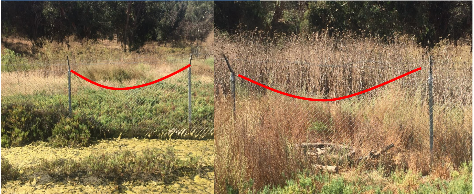
Fence lines bent and warped down
