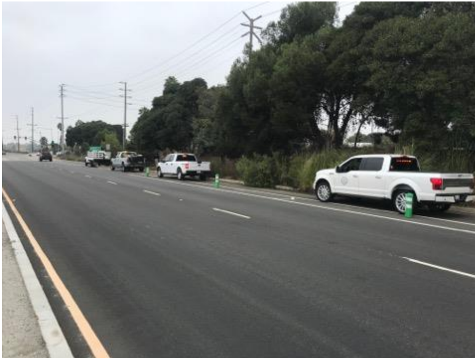
The vegetation on the property is growing out onto the street causing anyone riding in the bike lane to transverse out into the traffic lane, a major liability. Also notice we have an on going water leak coming off the property.
