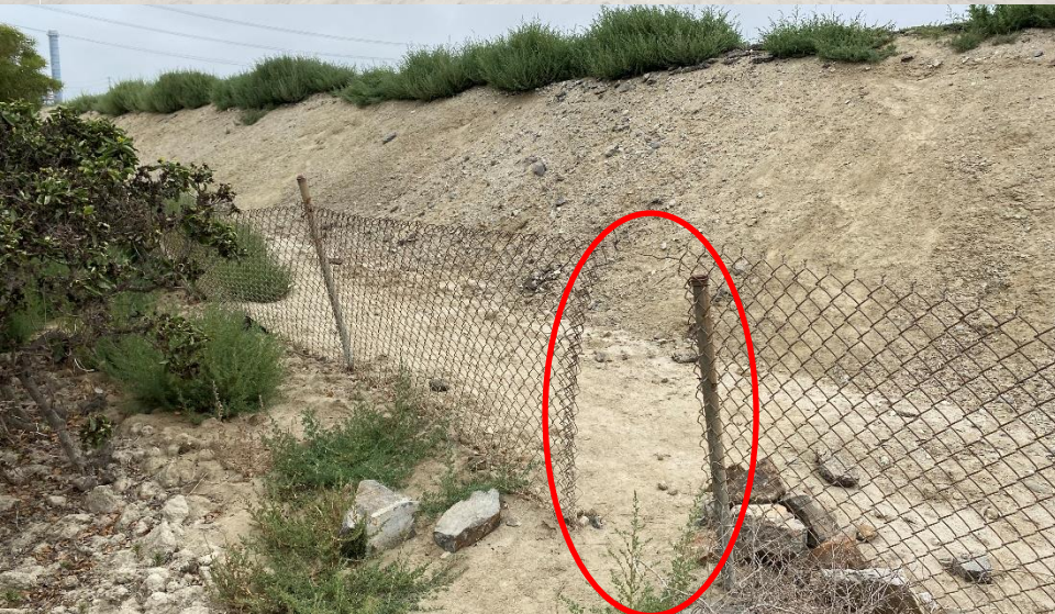
Fence breach along eastern fence line
