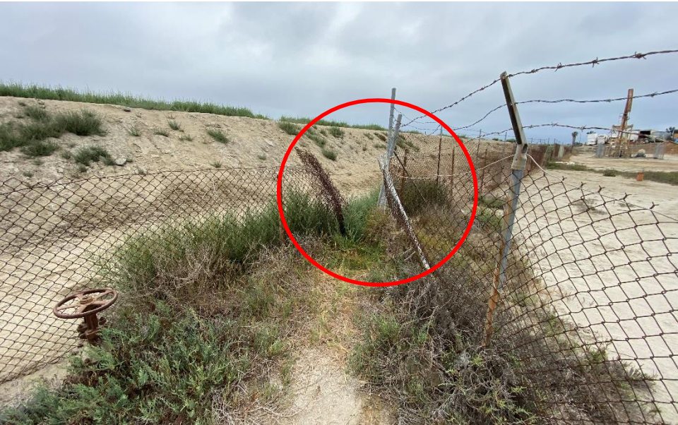
Fence breach in southeast corner of property
