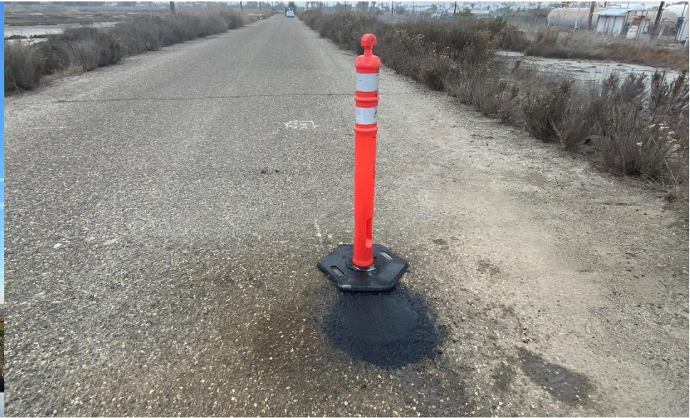
Borings conducted along road and refilled
