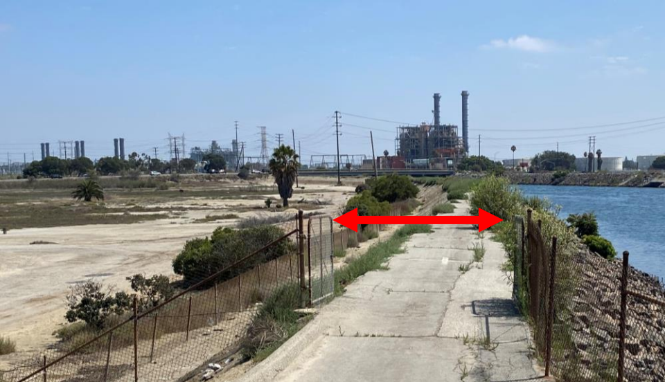
Levee gates left open
