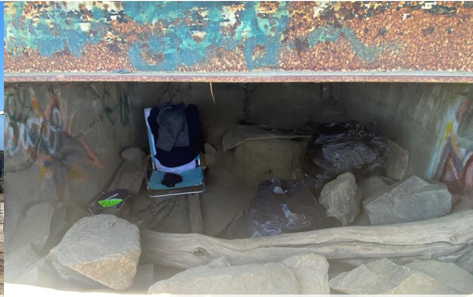
Materials under bridge
