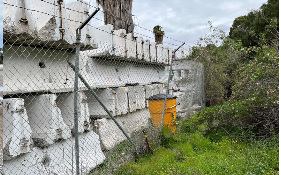
Fence line portion that lessee has replaced
