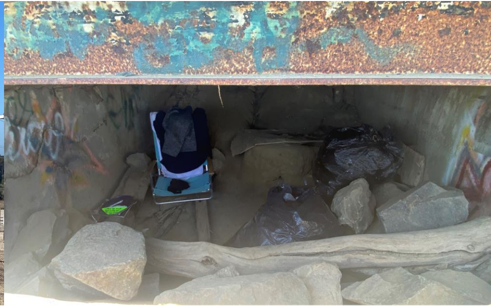
Materials under bridge
