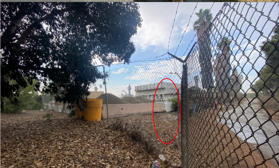
Fence line breach in southeast corner
