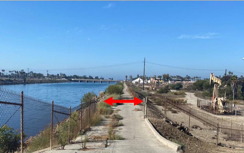
Levee gates found open
