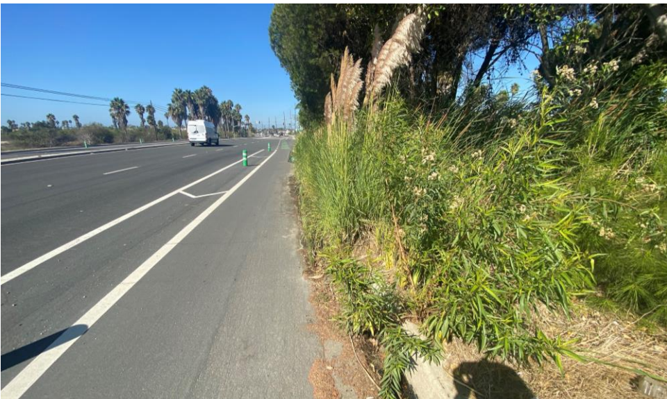
Vegetation encroaching bike path
