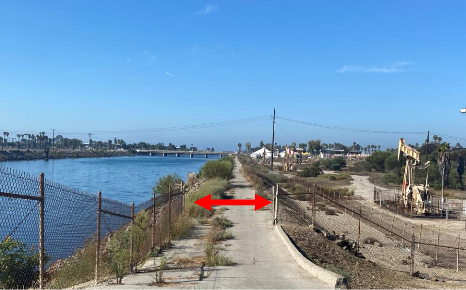
Levee gates found open
