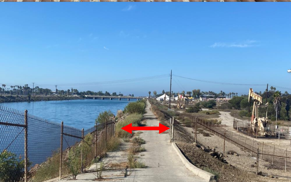
Levee gates found open
