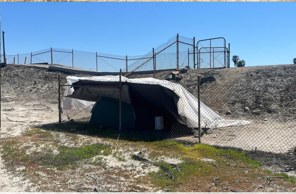
Encampment next to levee
