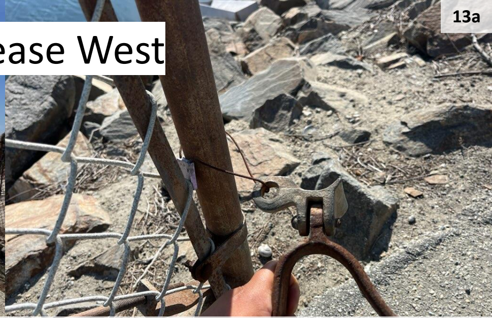
Southern levee gate damaged and open
