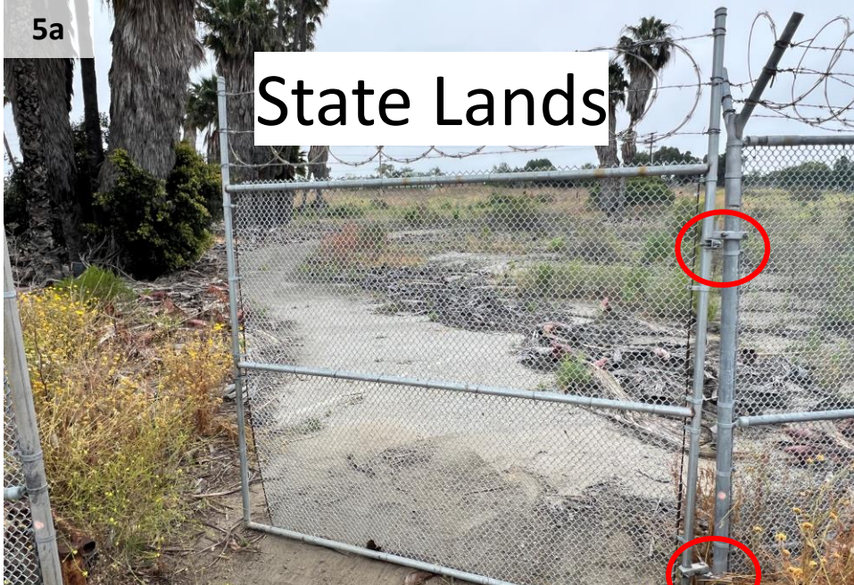
Damaged gate hinges
