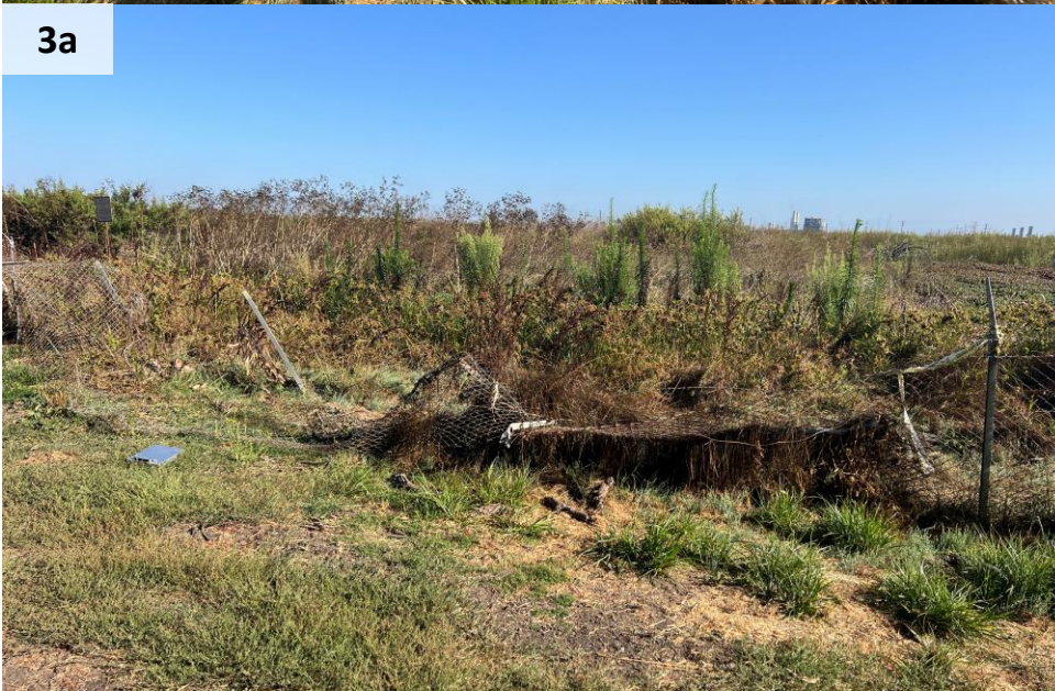
Damaged fence near Gum Grove Park entrance
