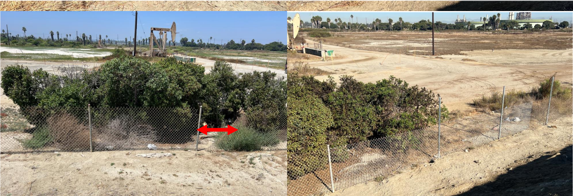
Fence breach repaired
