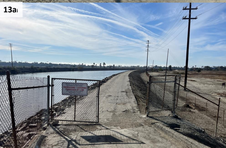
2 nd Street levee access gate open
