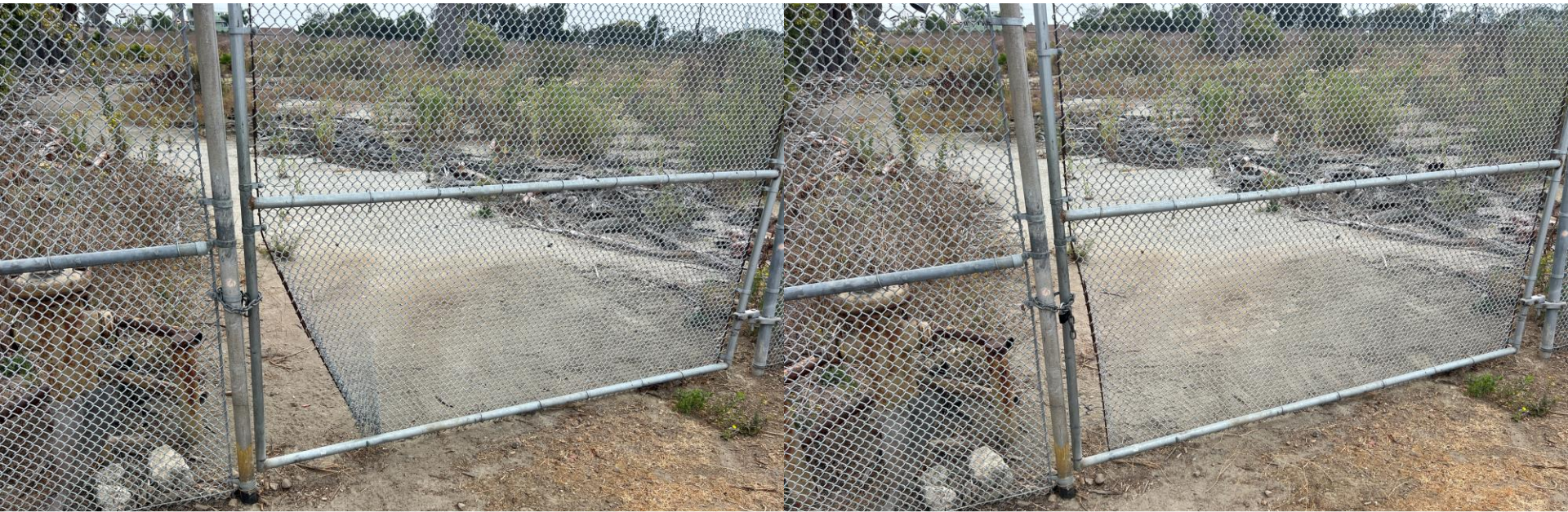
Fence breach repaired
