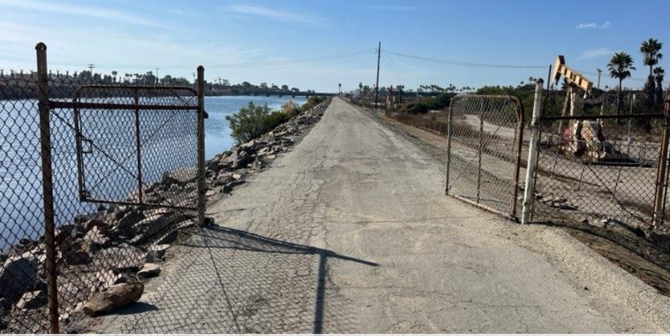
Southern levee gate damaged and open
