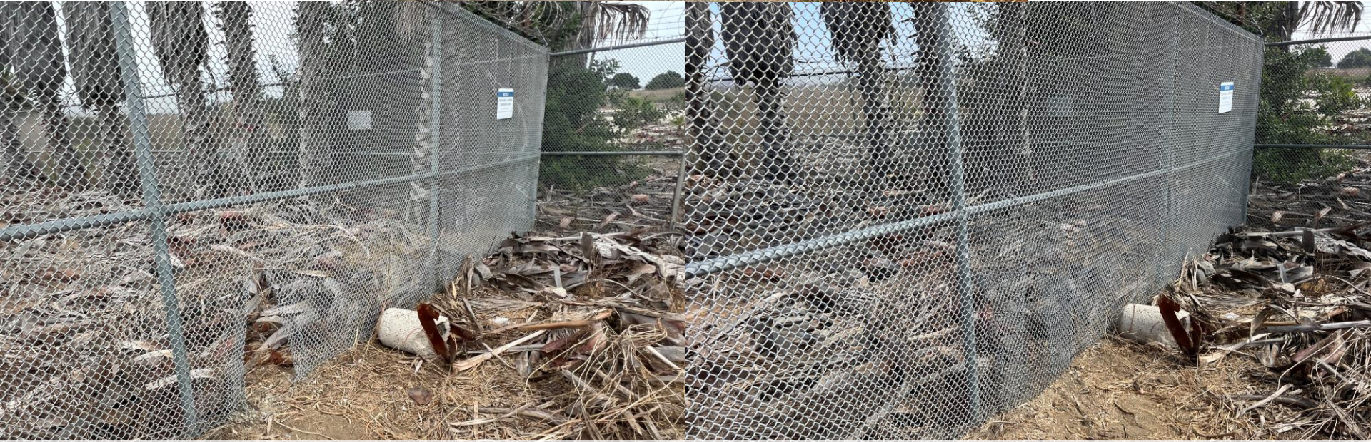
Fence breach repaired
