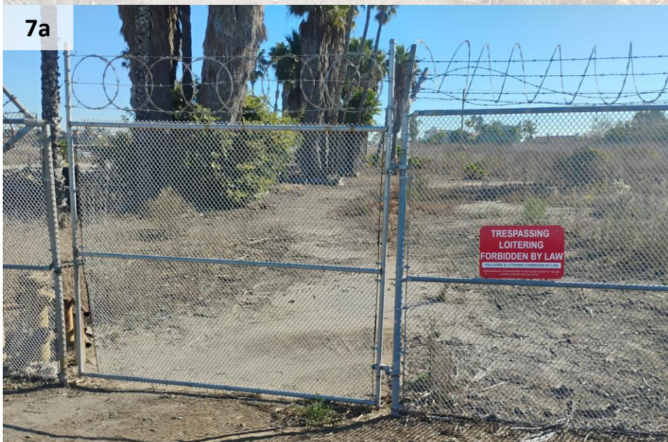
"No Trespassing" sign installation
