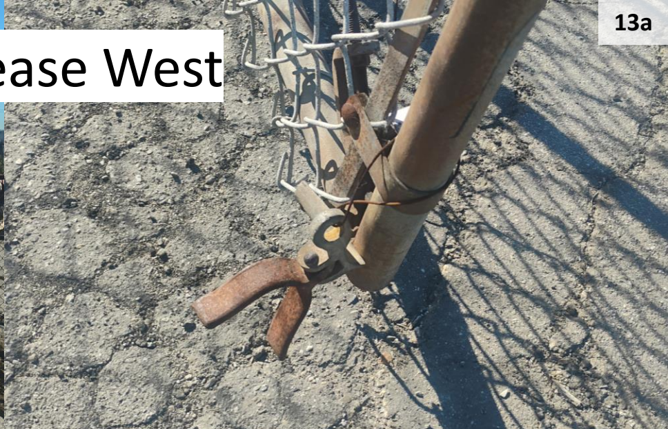
Levee gate damaged and open
