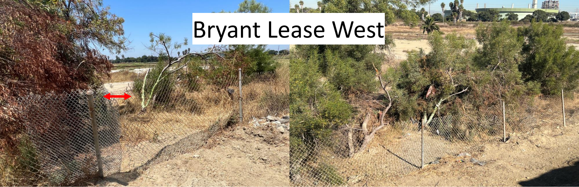
Fence breach repaired
