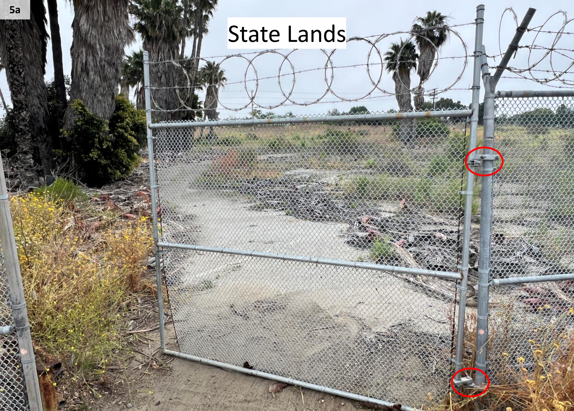
Damaged gate hinges
