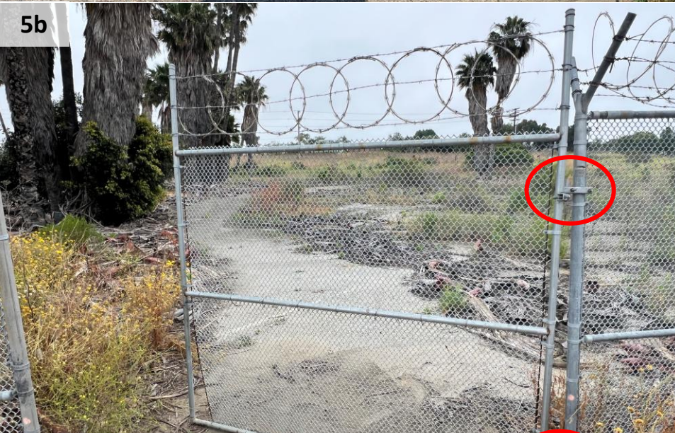
Damaged gate hinges
