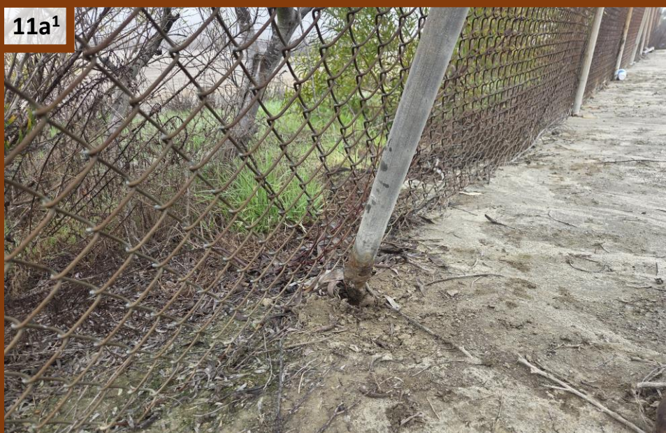
Fencepost loose due to continued soil erosion.
