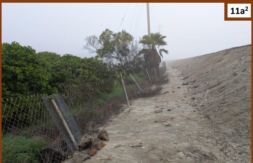
Fencepost loose due to continued soil erosion.
