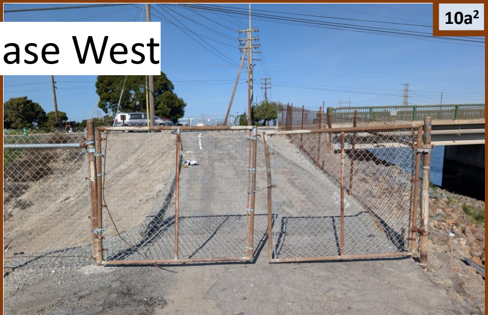
2 nd Street SGR levee access gate repaired and locked.
