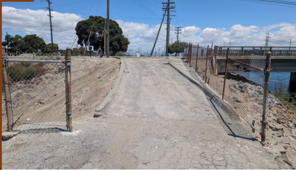
2 nd Street SGR levee access gate has been removed.
