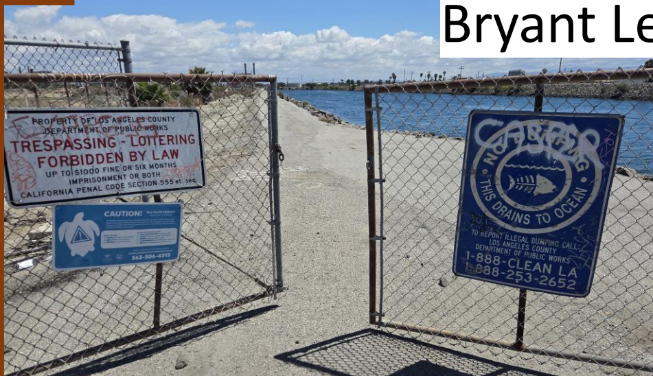
PCH SGR levee gate unlocked and open.
