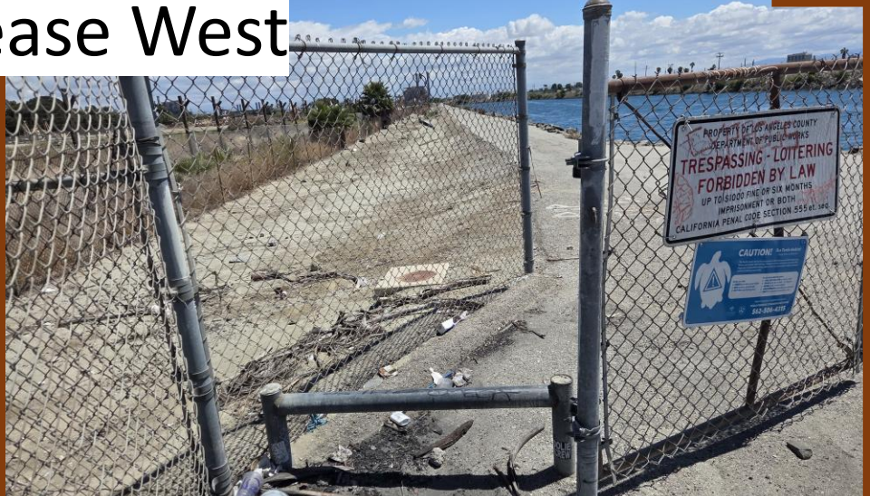
PCH SGR levee gate open.
